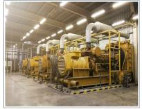
Fig. 170: Diesel-operated emergency generator
