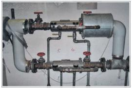
Fig. 81: Filter system (redundant design)
