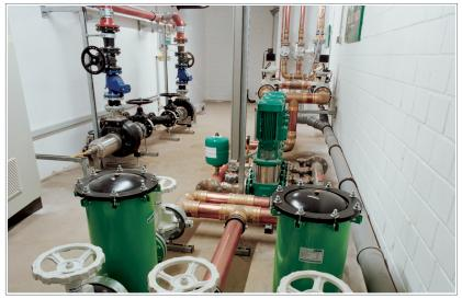
Fig. 100: Viega piping system Sanpress XL in a water treatment plant
