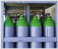
Fig. 147: Secured liquid gas cylinders
